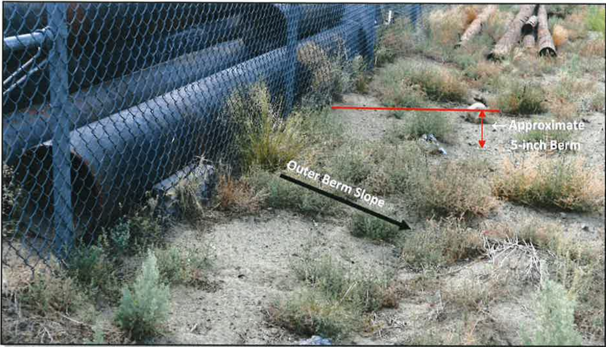
Figure 8: Outside of North Fence showing an approximate 5-inch berm.
