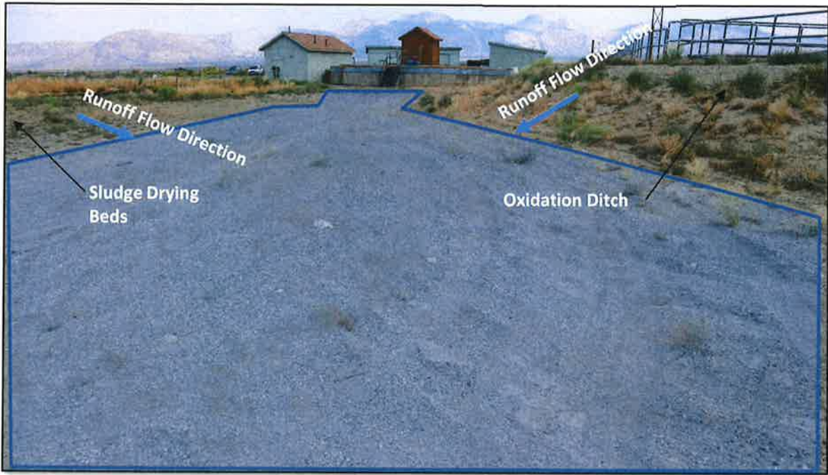
Figure 10: Depression Area (In Blue) Between Oxidation Pond and Drying Beds.
