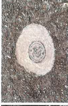
Snowplow damage mended
