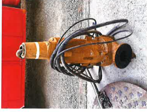
Old pumps pulled
