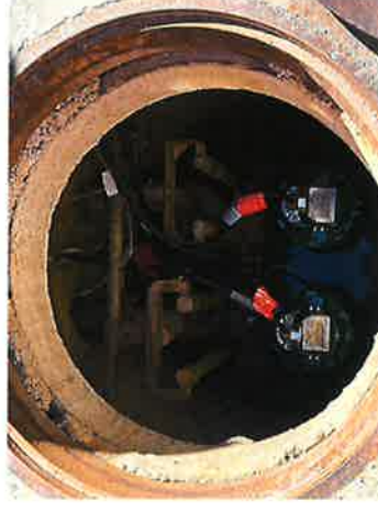
New pumps installed
