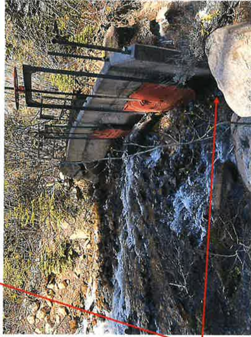
Location of dam undermining
